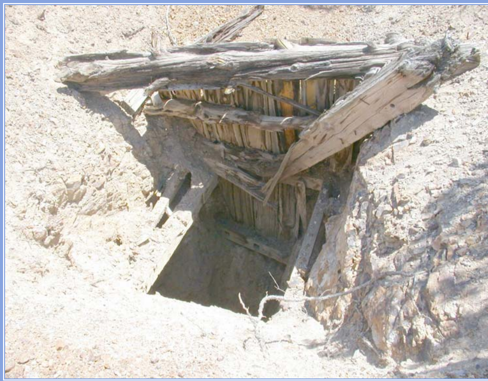
Dangerous Vertical Openings at Cerrillos Mine Safeguard Project. (Both Opening are High Priority Hazards)
