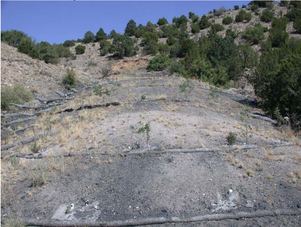
Madrid Reclamation Project – Post-Reclamation Terrace / Stabilization of Coal Waste Pile.
