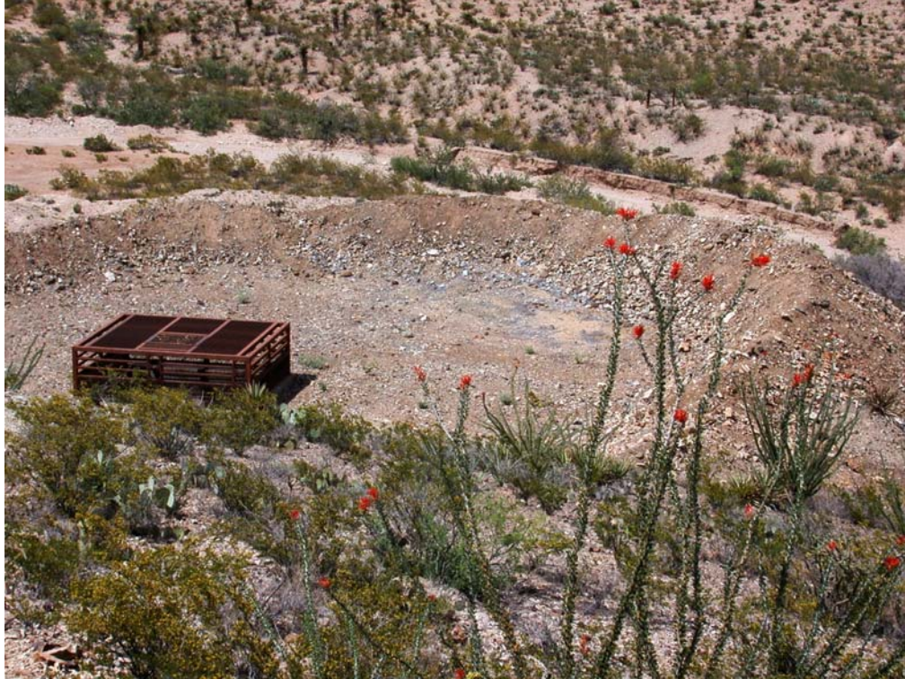
Orogrande Safeguard Reclamation Project – Berm used to control runoff and also serves to hide the bat cupola from view of visitors on the roads below.
