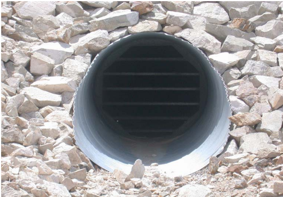
Bat gate in corrugated steel pipe at Orogrande Mine Safeguard Project.
