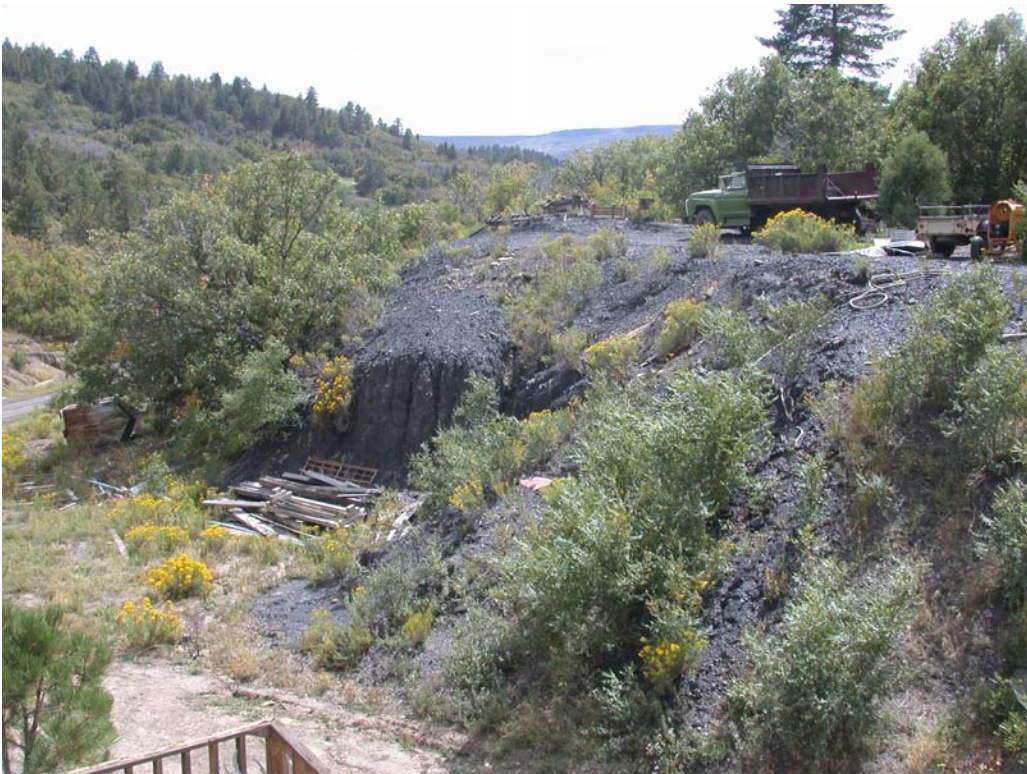
Yankee-Vukonich Gob Reclamation Project (pre-construction).
