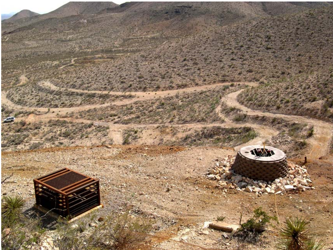
Orogrande Safeguard Reclamation Project - Garnet Mine (Post-construction).
