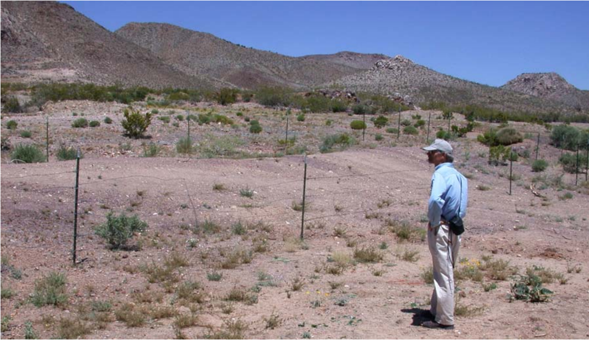
New Mexico Engineer John Kretzman Inspects for Settling at Flourite Ridge Reclamation Project. A Large Vertical Opening Was Backfilled At This Site. The Area Was Also Fenced Off For Additional Protection.
