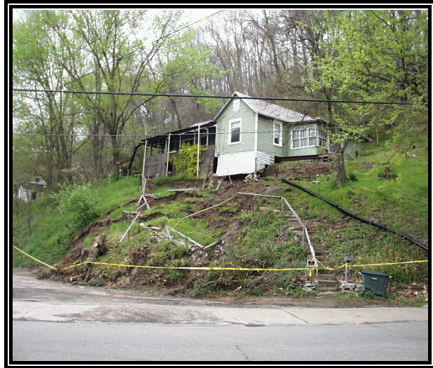
AML landslide impacting a house in Meigs County
