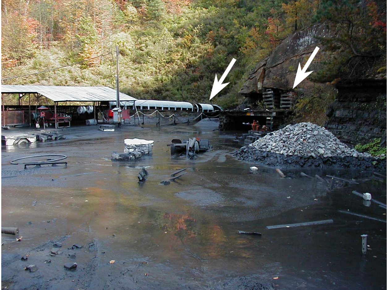
Photo 4. Number 2 North Portals - October 16, 2000. Source: OSM.
