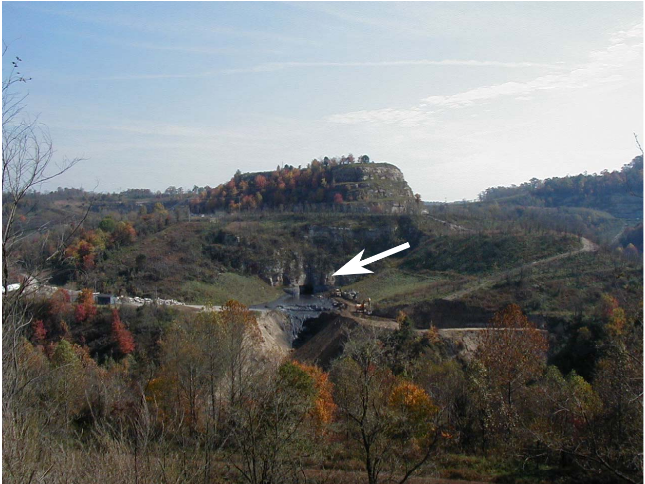
Photo 5. South Mains Portal - October 16, 2000. Source: OSM.
