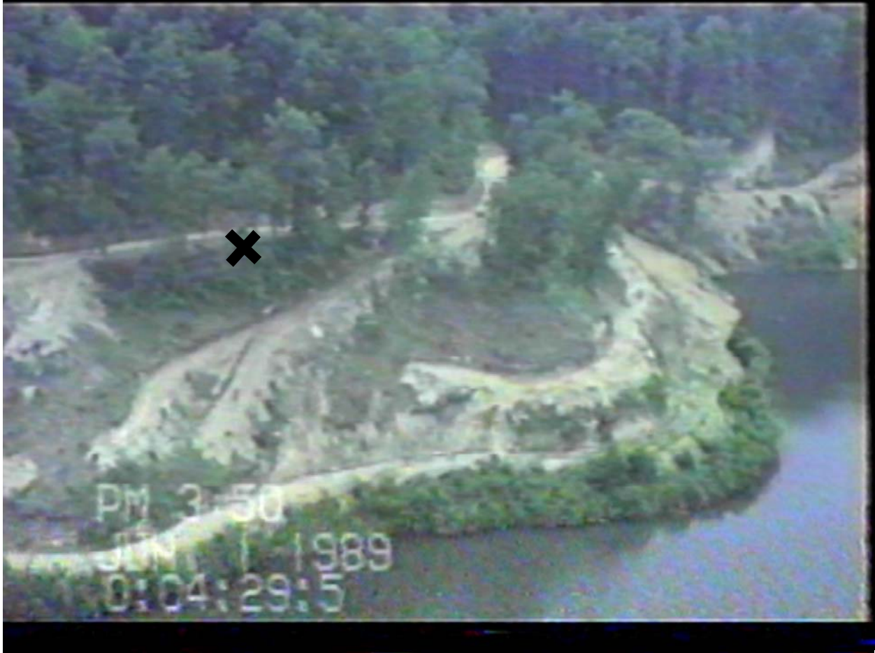
Photo 7. Surface Conditions at 1994 Breakthrough - June 1, 1989. Source: DSMRE aerial video. The X marks the approximate location of the 1994 breakthrough. Pool elevation 958 feet msl. Mine roof elevation 964 feet msl.
