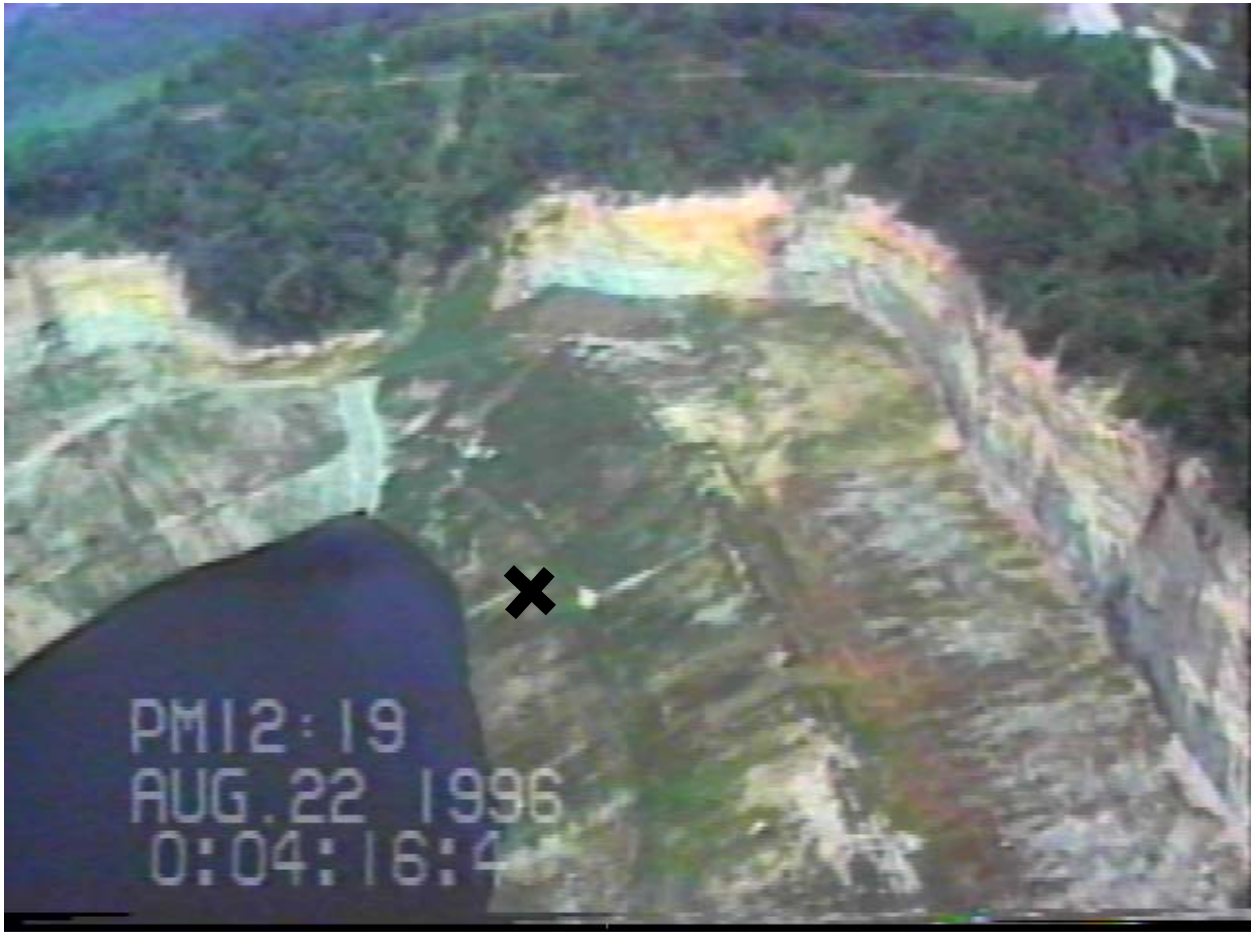
Photo 6. Seepage Barrier by 2000 Breakthrough (After Construction) - August 22, 1996. Source: DSMRE aerial video. The X marks the approximate location of the 2000 breakthrough. Pool elevation 1,018 feet msl. Mine roof elevation 973 feet msl. Contour bench elevation 1,075 feet msl.
