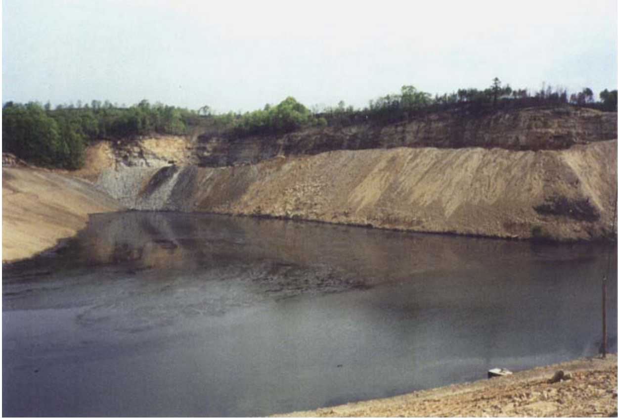
Photo 13. Seepage Barrier by 2000 Breakthrough (During Construction) - June 8, 1995. Source: GAI. The 2000 breakthrough area is located at the left-center of the photo. Pool elevation 1,001 feet msl. Mine roof elevation 973 feet msl.
