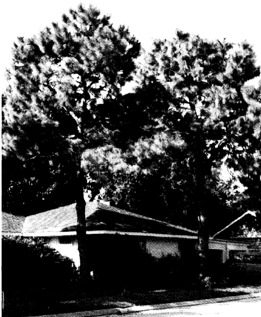
Figure 9-9—Twenty- to twenty-five-year-old loblolly pines providing shade and beauty in a south Louisiana suburb. The few needles deposited on the roof will be swept away with the next wind. The house has no gutters, so that clogging with needles is not a problem.
