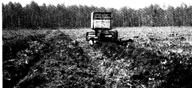
Figure 4-4 —Bedding a forest site with a crawler tractor and bedding harrow. Because the beds are not being packed, the soil should be allowed to settle for at least 6 months before planting bareroot seedlings.
