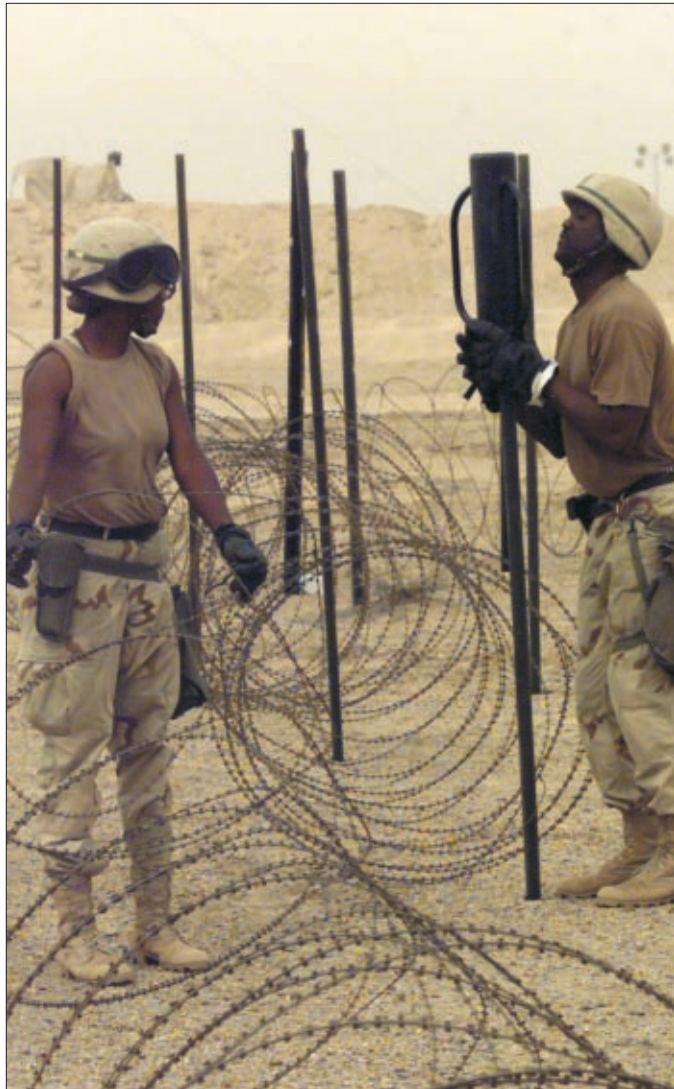
Sgt. 1st Class Alfonzie Brown of Moorehaven, Fla., pounds a picket as Spec. Yolanda Isaac, a physical therapist in Fort Lauderdale, Fla., waits at the ready with a coil of concertina wire.
