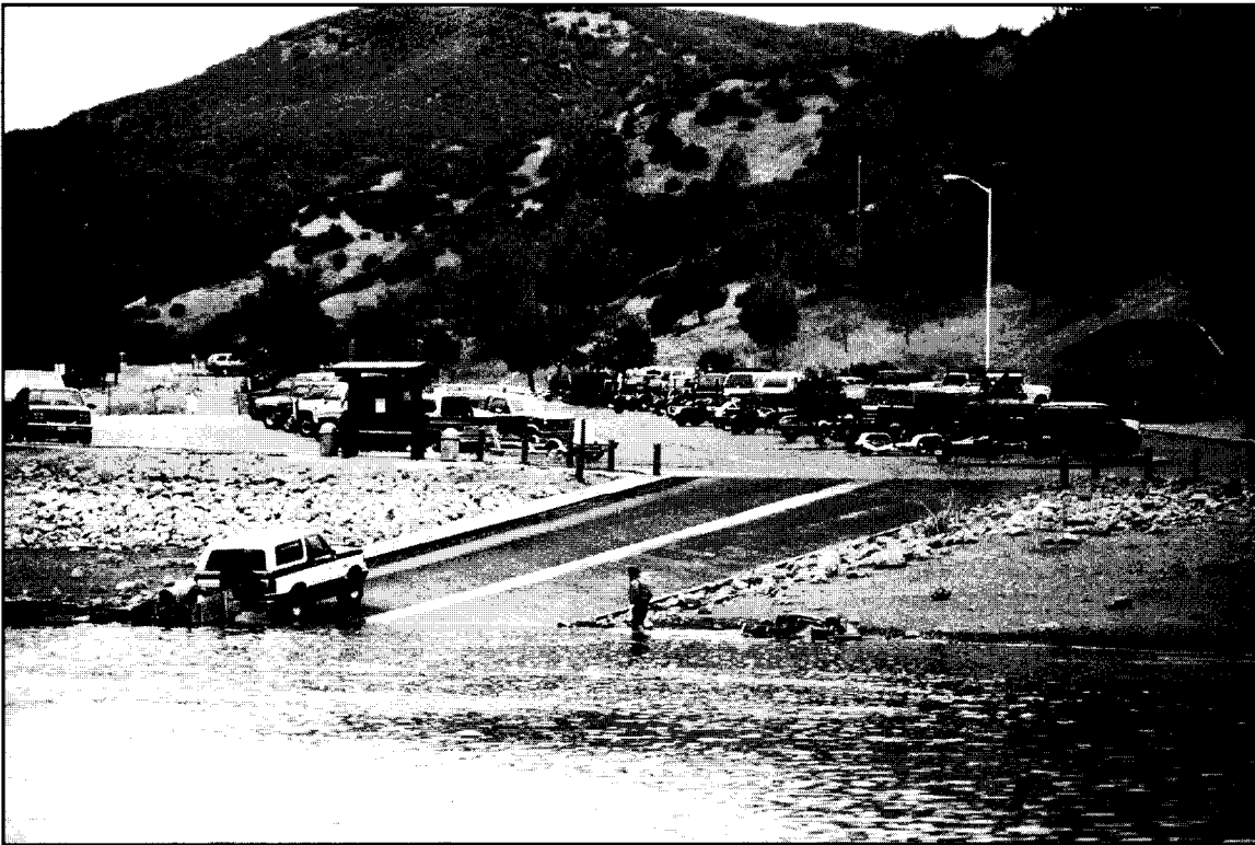
The Bureau of Reclamation is a major provider of water-based recreation facilities, including this boat ramp at Lake Berryessa, California.
