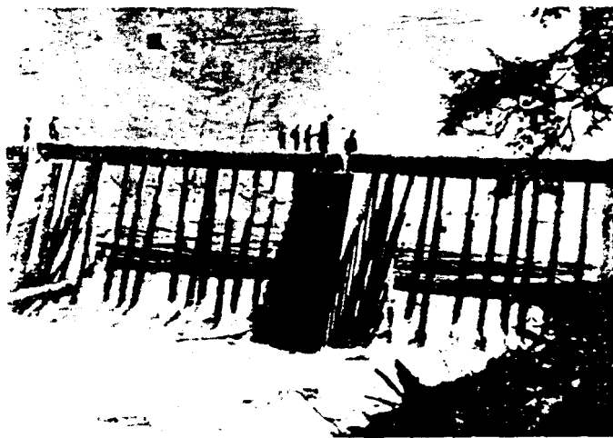
Figure 1. - Splash dam erected about 1910 on the Russell Fork Big Sandy River, Southwest Virginia.
