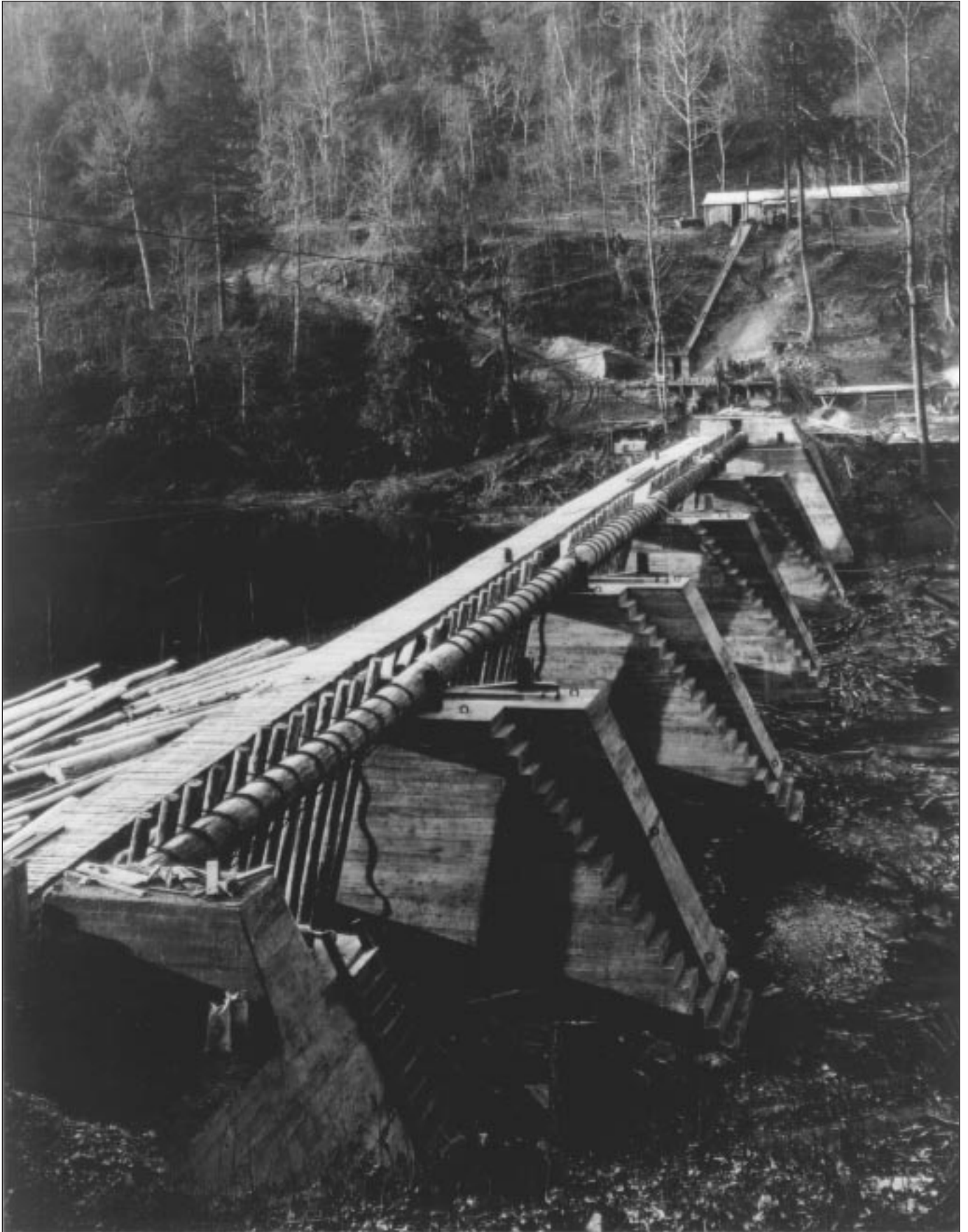
Figure 13—Great splash dam of the Yellow Poplar Lumber Company on the Big Sandy River, Virginia.
