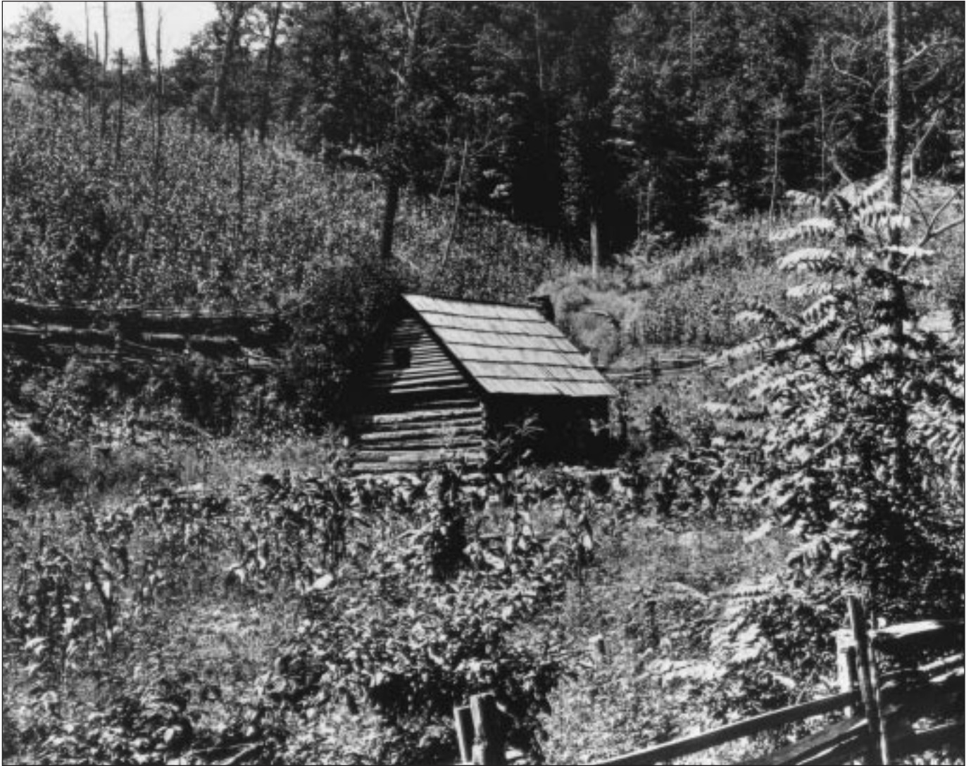
Figure 8—Typical mountaineer's cabin near Junaluska Mountain.
