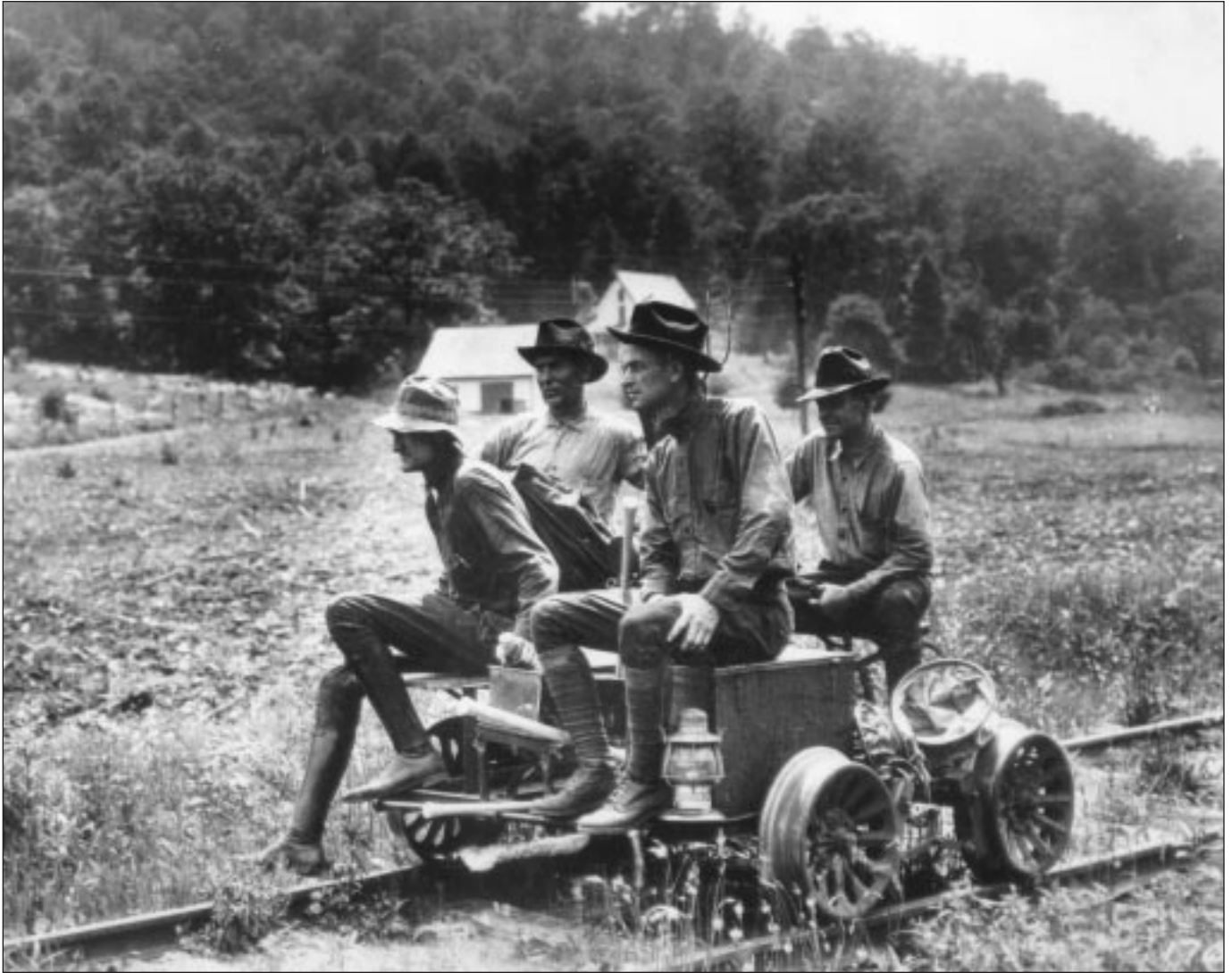
Figure 16—Pisgah National Forest crew riding to fire.
