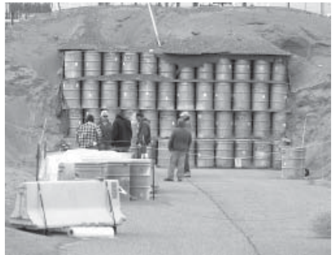
The front portion of buried drums containing waste is exposed in a trench at the Hanford Site.
