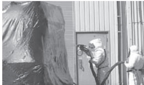
Rocky Flats workers encase equipment with InstaCote™ for shipment.
