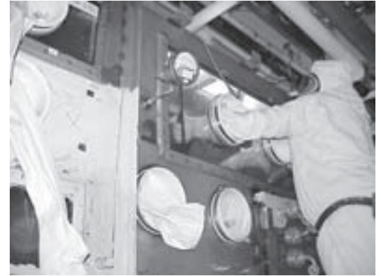
A worker applies decontamination solution to the inside of a Rocky Flats glove box.
