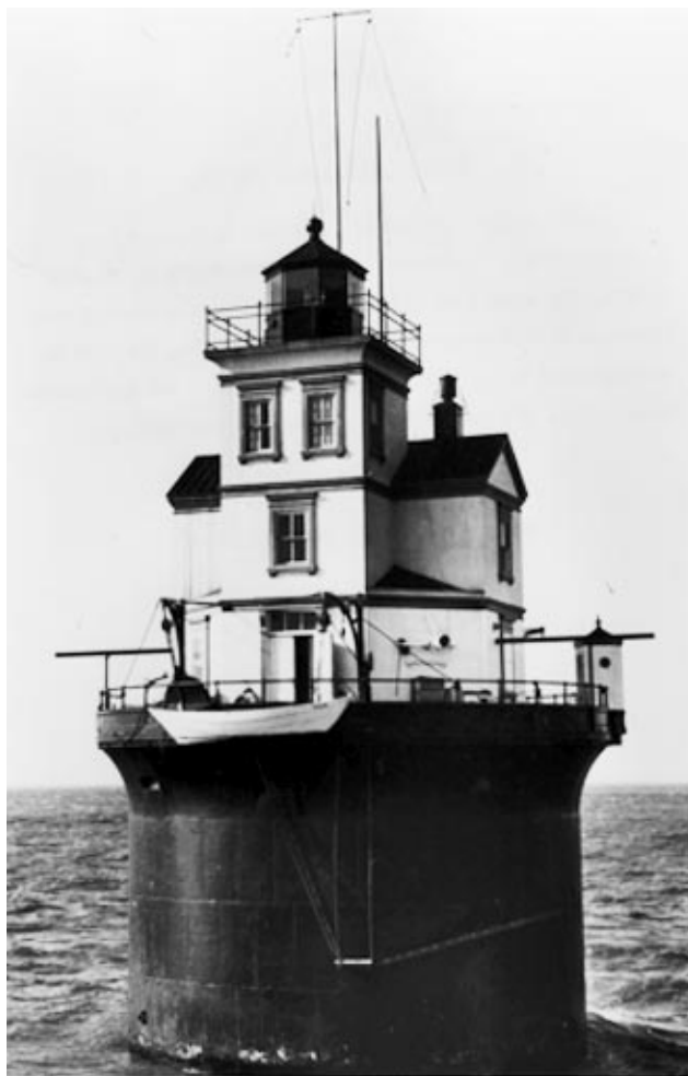
Fourteen Ft. Bank Light in Delaware Bay. Note differences in appearance with Miah Maull shown earlier. Official U.S. Coast Guard Photograph.
