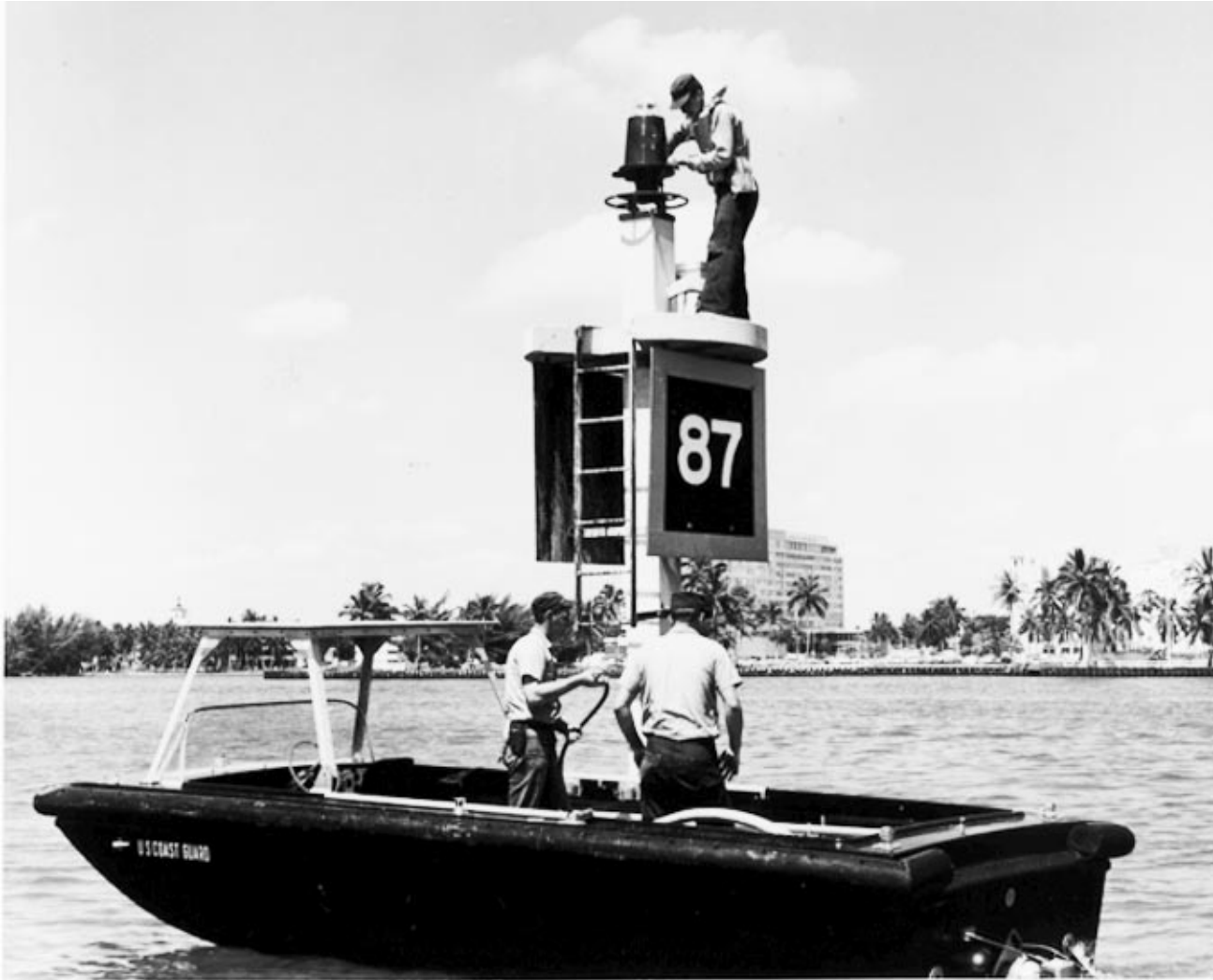
U. S. Coast Guard ATON personnel servicing daymark and light, Miami, Florida. Official U.S. Coast Guard Photograph
