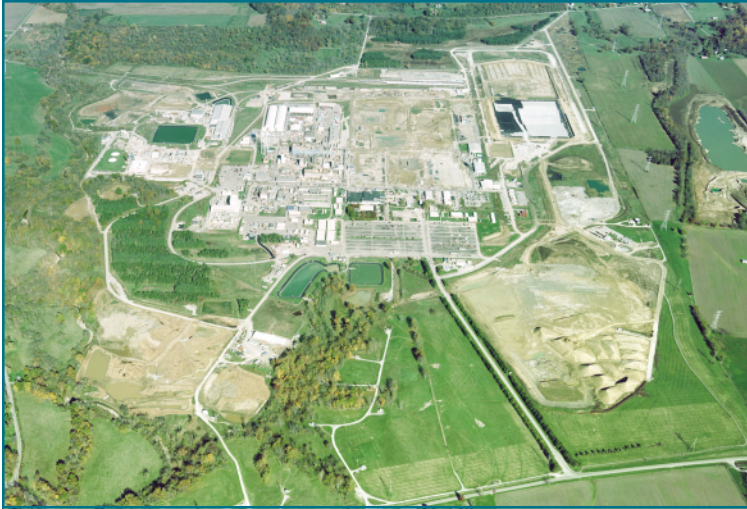
Figure 41. Aerial view of the Fernald FMPC.
