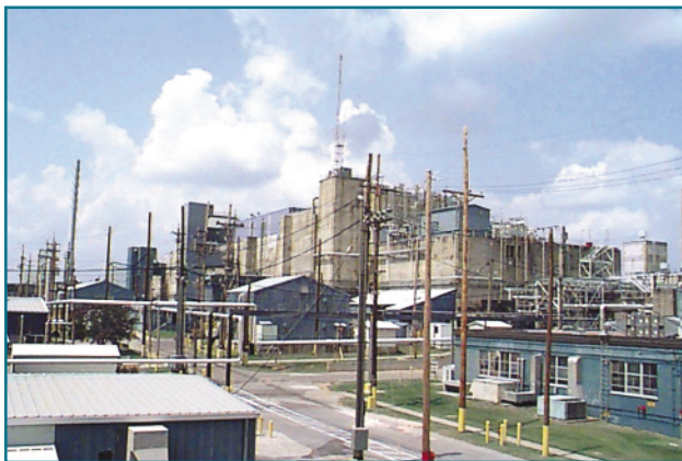
Figure 14. F-Area Canyon Facility recovered uranium from targets.
