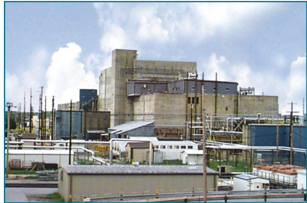
Figure 15. H-Area Canyon Facility (221-H Building) recovered uranium from enriched driver fuel.
