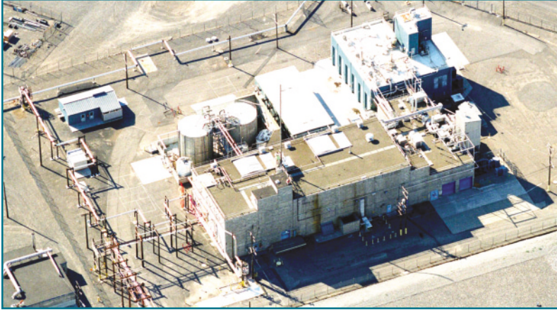
Figure 9. Aerial view of the UO_3 Plant at Hanford Site, which processed about 80% of the recycled uranium shipped.
