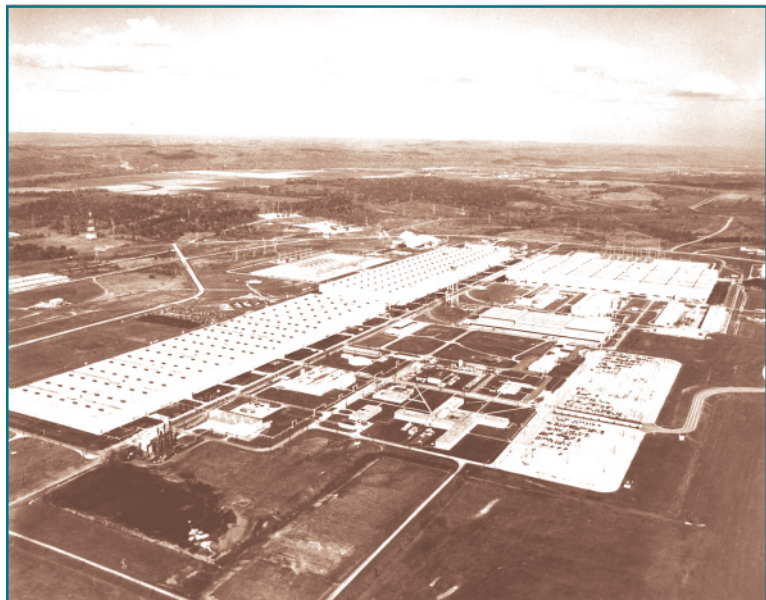
Figure 37. Aerial view of the Portsmouth Gaseous Diffusion Plant.
