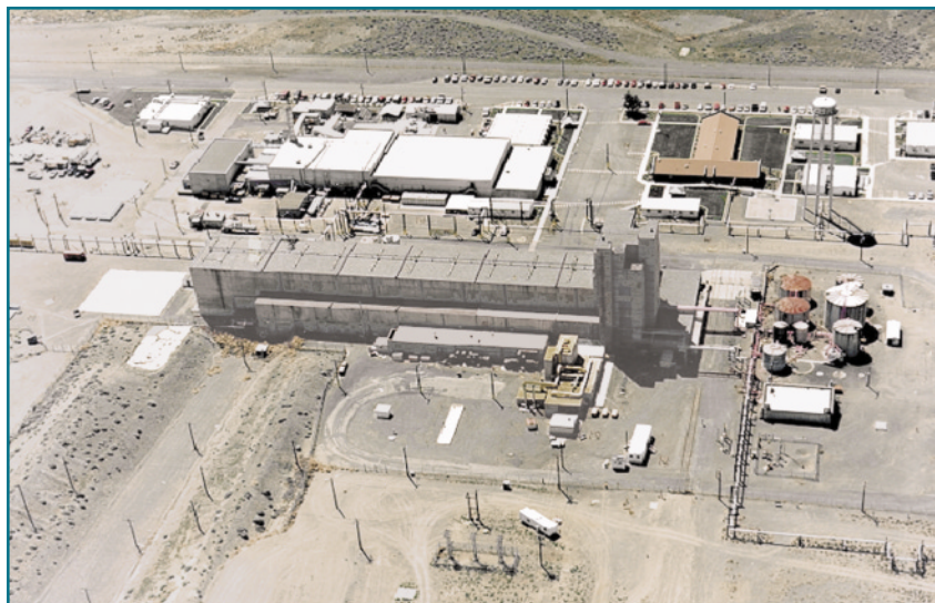
Figure 7. The Hanford REDOX Plant recovered uranium from spent fuel from 1952–1967.
