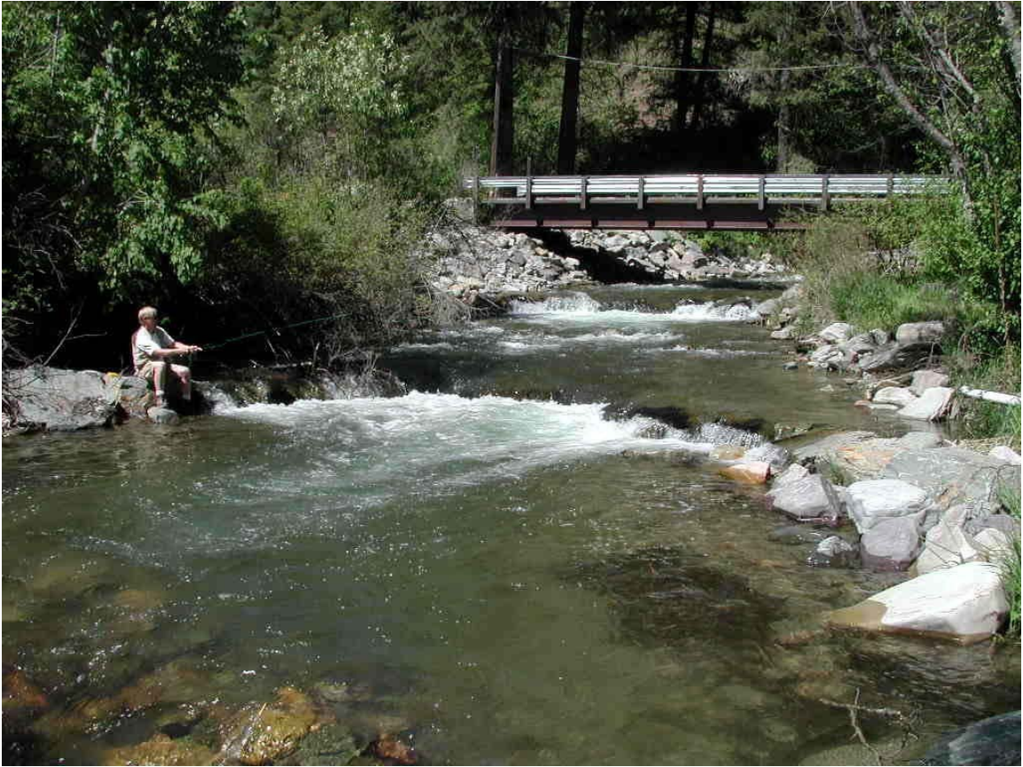
Figure 46. O'Brien Delta Project photo showing cross-vanes and new bridge.
