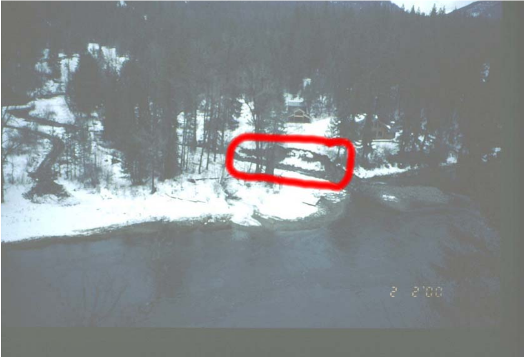
Figure 45. O'Brien Creek Delta Project site with eroded bank highlighted.
