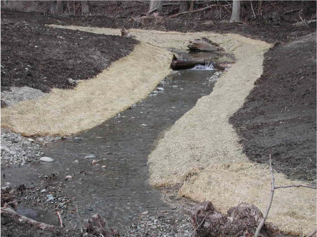
Figure 26. Sinclair Creek, shortly after the channel reconstruction work completed in 2001.
