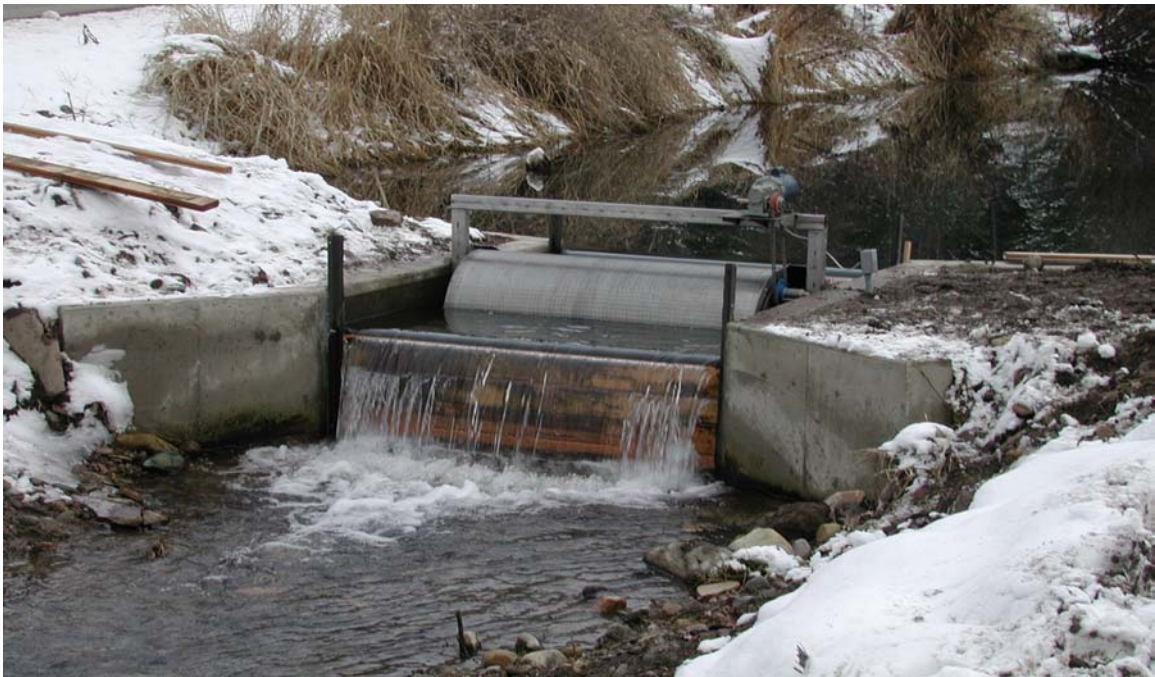
Figure 52. Fish screen at Libby Field Station spring pond, Libby, MT.
