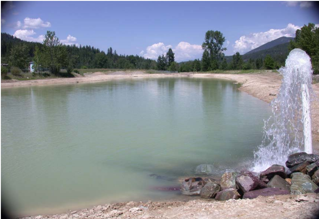
Figure 1. A photograph of the Troy fishing pond shortly after construction during the 2002 summer. The maximum depth is 17 feet and total area is approximately 2 acres. Landscaping will be completed by the City of Troy. The pond has been successfully stocked with rainbow trout produced by Montana FWP at the Murray Spring Fish Hatchery in Eureka, MT.
