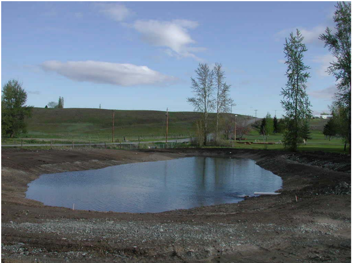
Figure 2. A photograph of the Eureka fishing pond taken shortly after construction. The pond has a maximum depth is 8 feet and a total surface area of 0.4 acres. Fish stocking has been delayed until the pond completely seals.
