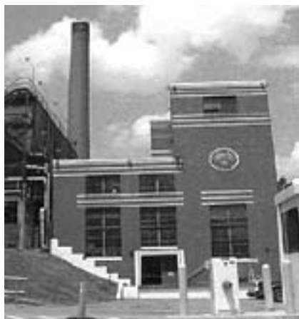
Figure 1. The NIOSH boiler plant was modified to cofire biomass with coal.
