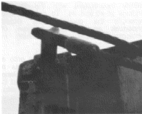
Twisted eye/hook connection
