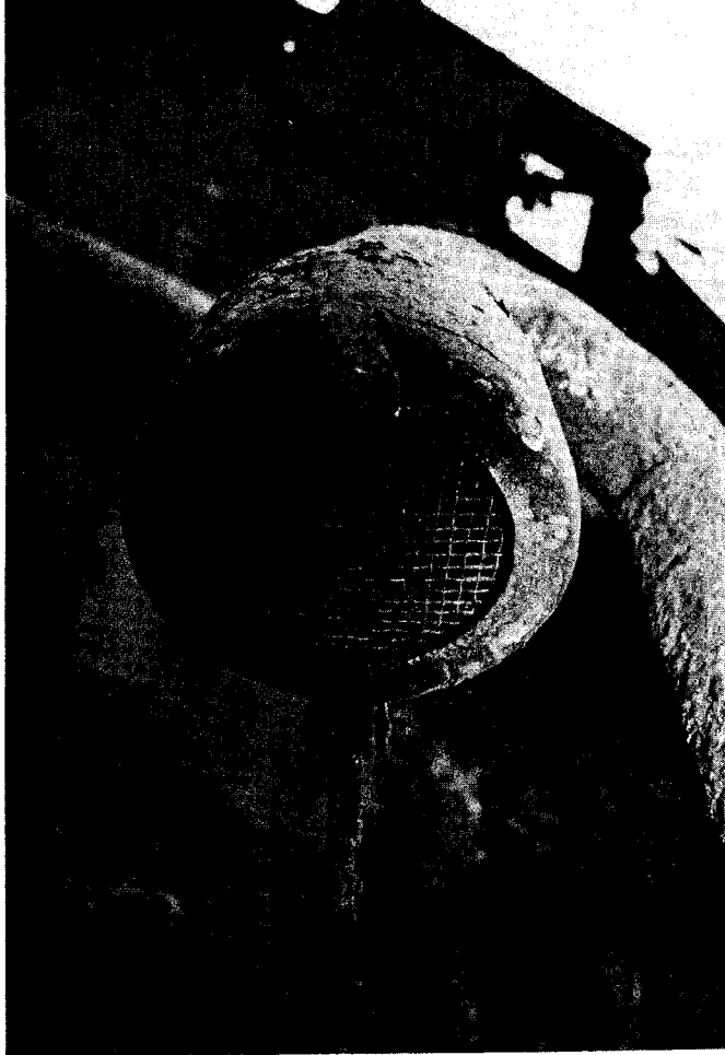
Picture of the aft vent for the starboard fuel oil (bunker) storage tank taken by a HIRI representative showing the gooseneck and flame screen assembly in place.
