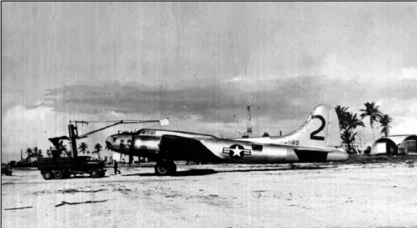
“Box” filter being removed from a B-17 “drone” cloud sampling aircraft
