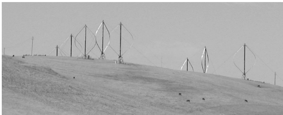
Figure 10: Vertical Axis Wind Turbines, Altamont Pass, California
