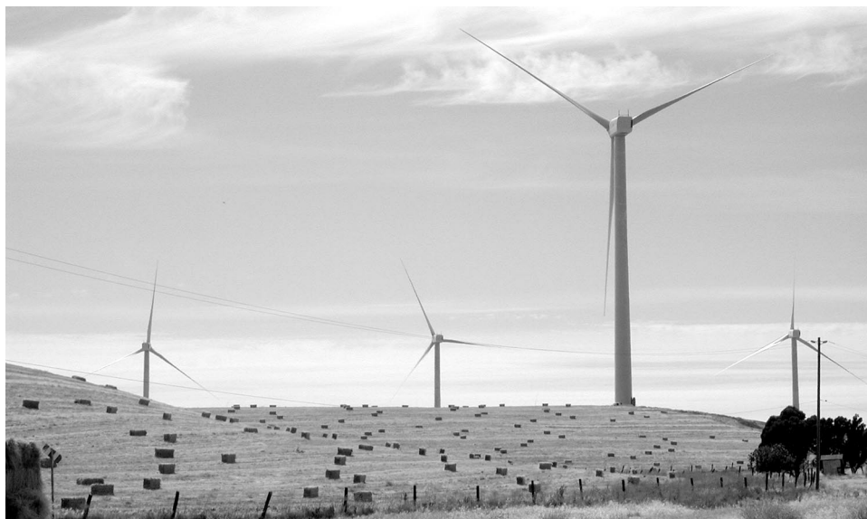
Figure 11: Wind Turbines, Solano County, California
