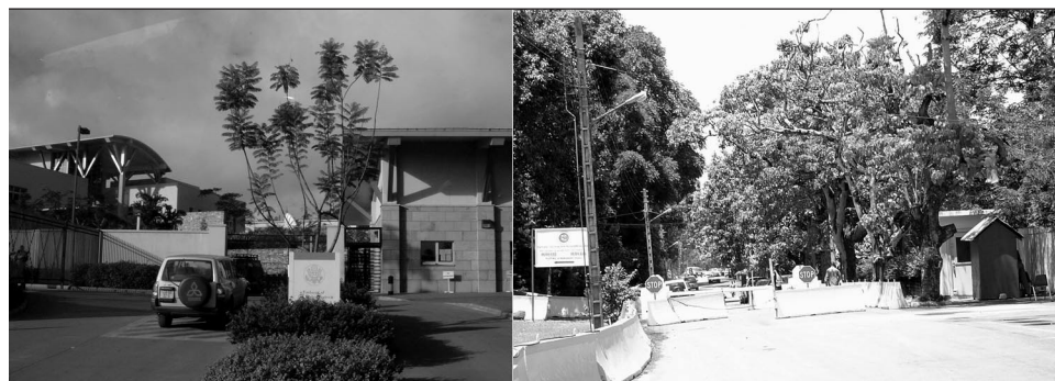
Figure 3: Hardened Access Facility at New Embassy Compound (left) Compared with USAID-Guarded Entrance in Same City
