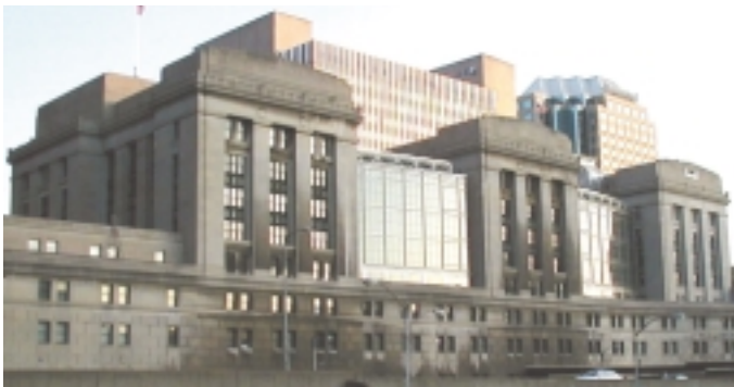
Window wells are being in-filled to provide space for additional courtrooms.
