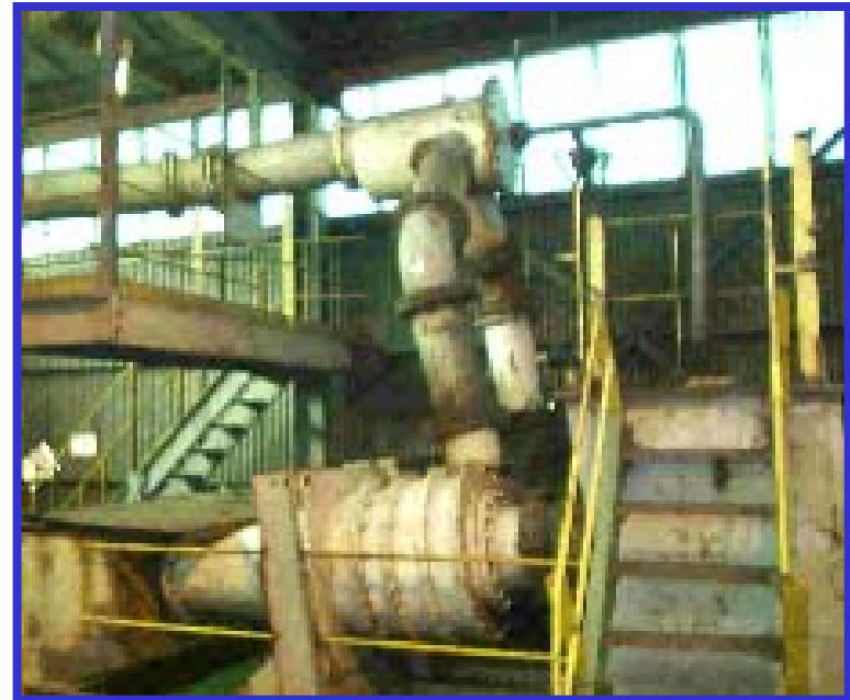
An installation of twin parallel coarse coal heavy media cyclones that were sampled in detail and evaluated using the density tracers .
