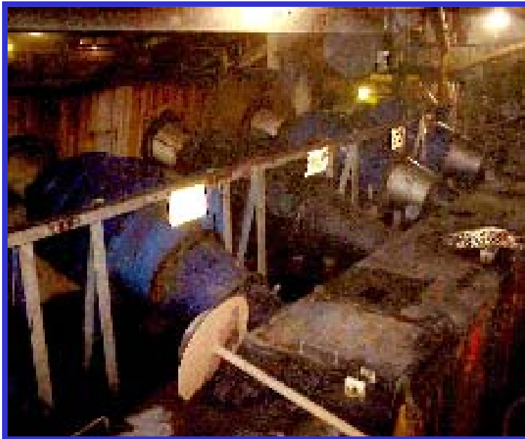
A bank of parallel coarse coal heavy media cyclones that were sampled in detail and evaluated using the density tracers .
