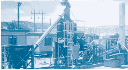
By-product recovery at a copper mine
