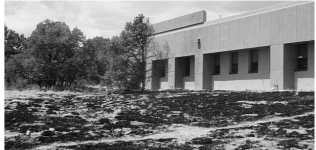
Wildfire scorched the grounds near Building 326 at Technical Area-46.
