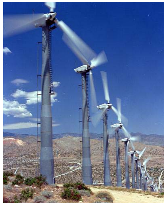
Photographs like this one from BLM's Wind Energy PEIS Web site ( http://windeis.anl.gov ) illustrate the siting of wind turbines in a desert landscape in western states.
