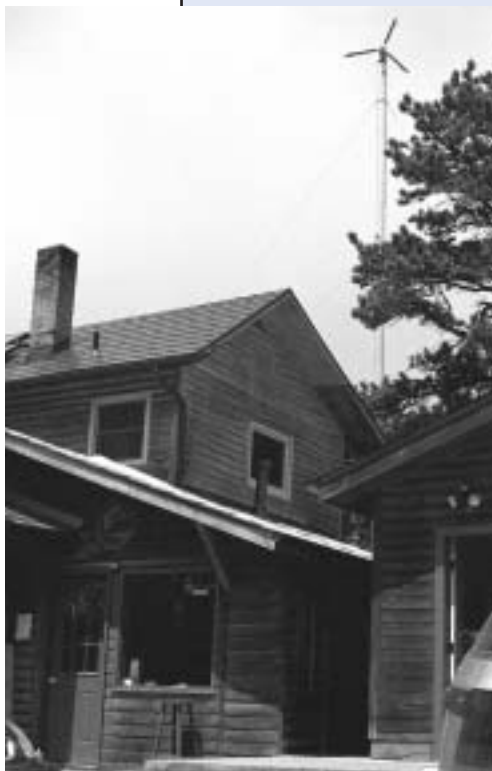
Jim Green, NREL / P1A12796
