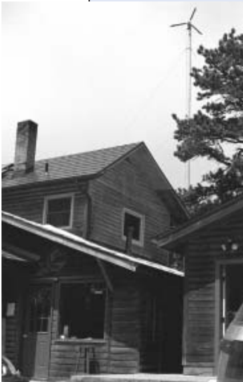
Jim Green, NREL / P1A12796
