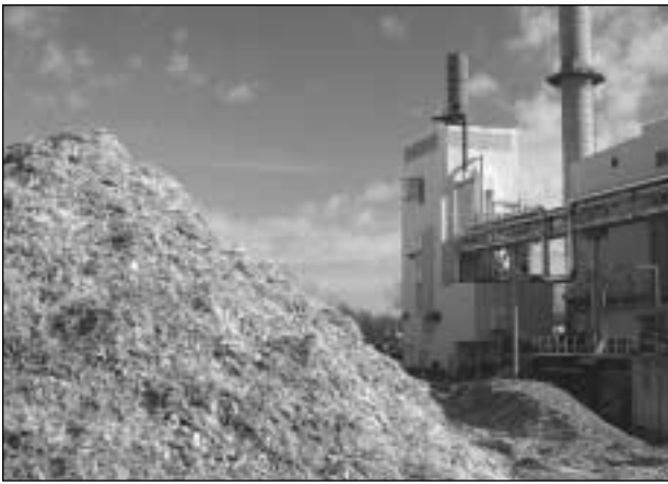
This gasifier in Burlington, Vermont, converts biomass into a clean gas for electricity production
