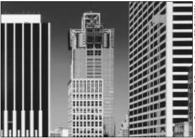
The Four Times Square Building in New York City uses thin-film PV panels to reduce the building's power load from the utility grid.
