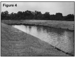
The flood control features suggested for the Hickory Creek included three different treatments of the creek banks. The banks were to be changed from their existing condition (Figure 1) to either a fabric-formed concrete embankment (Figure 2), a vertical concrete wall (Figure 3), or an earthen embankment (Figure 4). [Photos reprinted with permission from Environmental Impact Assessment Review, Vol. 17(4), Sullivan, W.C., F.E. Kuo and M. Prabhu, "Communicating with Citizens:
