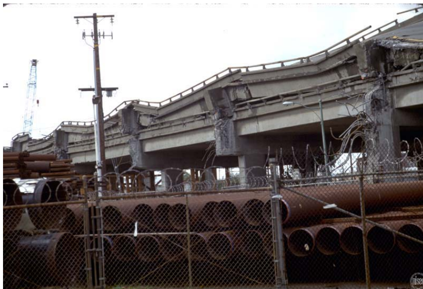
Figure 2.5 Collapse of the Cypress Avenue Freeway, 1989 Loma Prieta, California, earthquake. Reproduced courtesy of the National Information Service for Earthquake Engineering, University of California, Berkeley.
