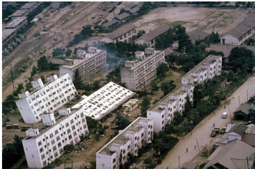
Figure 2.3 Foundation failures resulting from liquefaction, 1964 Niigata, Japan, earthquake. Reproduced courtesy of the National Information Service for Earthquake Engineering, University of California, Berkeley.
