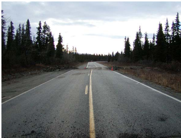
Figure 2.9. Lateral highway offset of 2.5 meters as a result of the 2002 Denali, Alaska, Earthquake. SOURCE: Alaska Division of Natural Resources.
