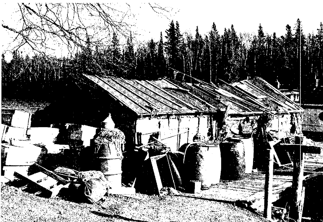
Fig. 6.18. Rear of fish house showing addition. The original structure, built of split logs is markedly different in construction than the rear portion using milled lumber. NPS photo by C. R. Humberger, 1949.
