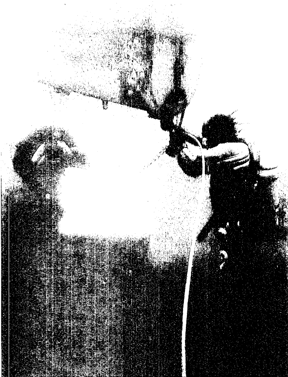
Fig. 7.7. "Underwater Mule" Park maintenance and protection staff designed this homemade lift apparatus to precisely place mooring buoy weights underwater. NPS photo by Joe Strykowski.
