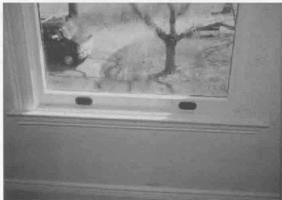
Typical Window Sash Condition After Restoration
