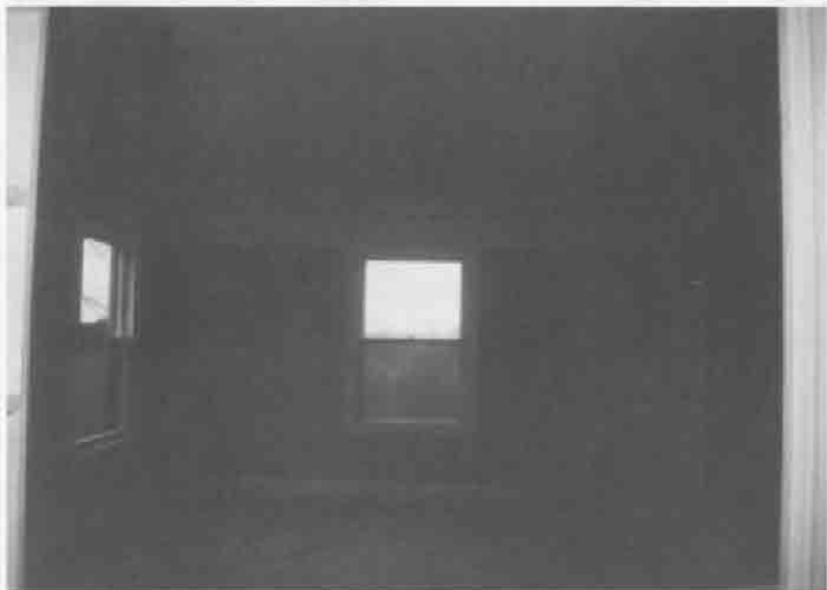
Gate Room: After Restoration
