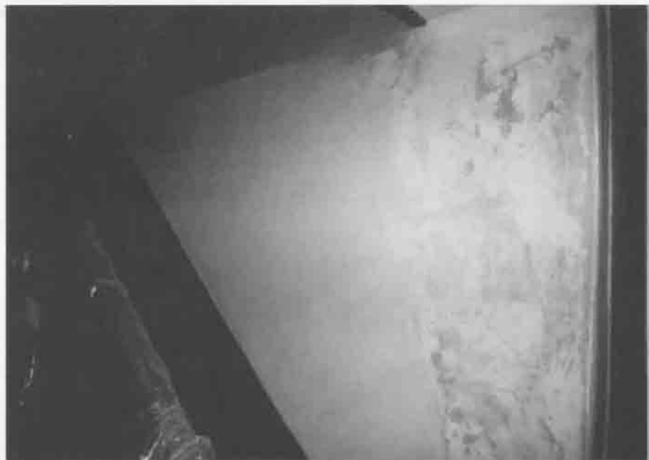
Second Floor Rear Hall Stairway: After Replastering
