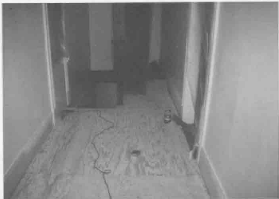
Third Floor Hall: Plywood Installed On Floor
