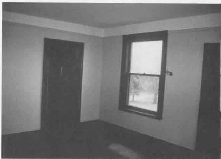
Nursery: After Restoration
