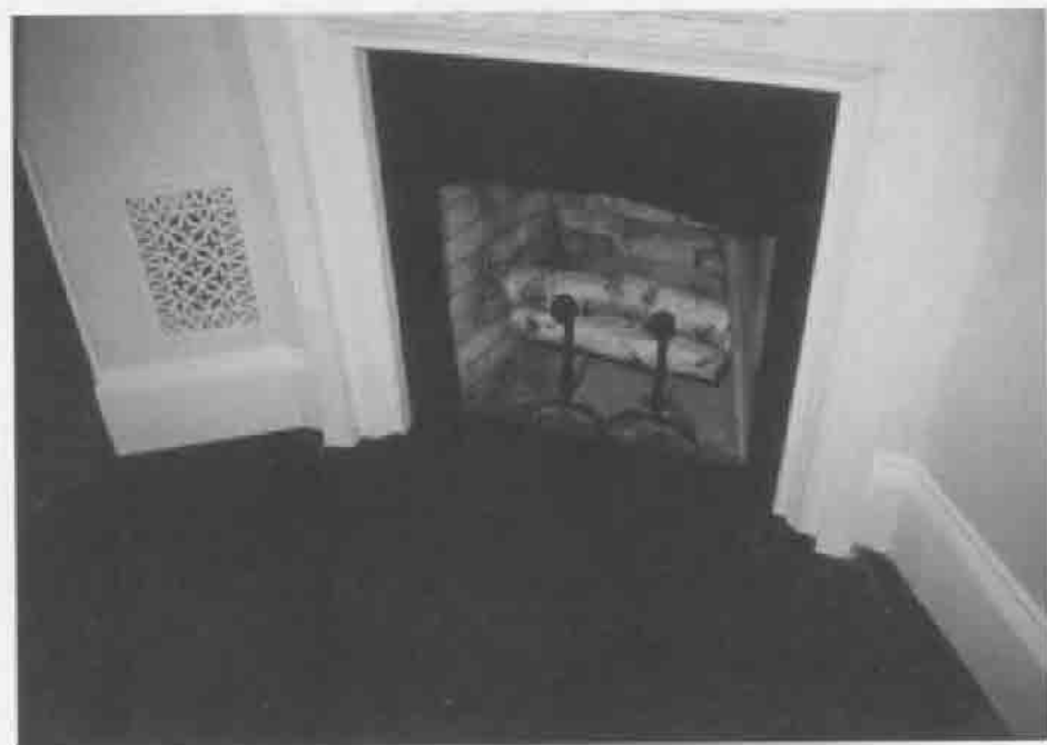
Mother's Room: Condition of Fireplace Hearth After Relaying, Repointing, and Repainting
