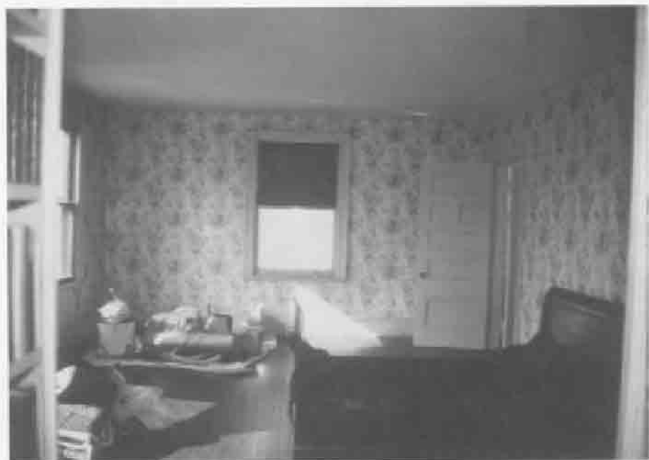
Gate Room: Before Restoration
