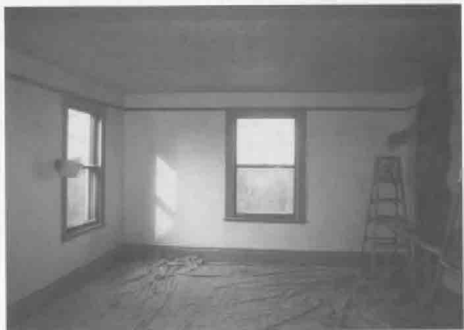
Gate Room: During Restoration (picture molding lowered, wallpaper removed).
