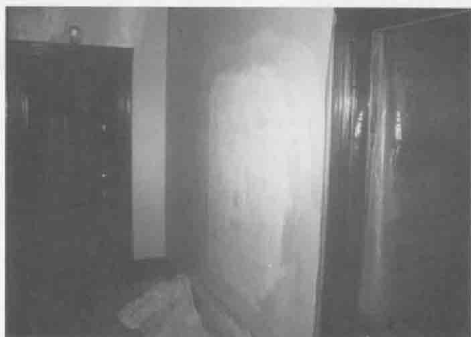
Typical Firebox Location After Removal and Replastering
