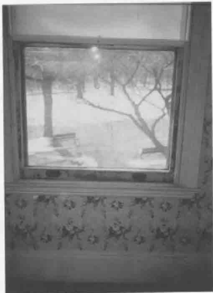
Typical Window Sash Condition Before Restoration
