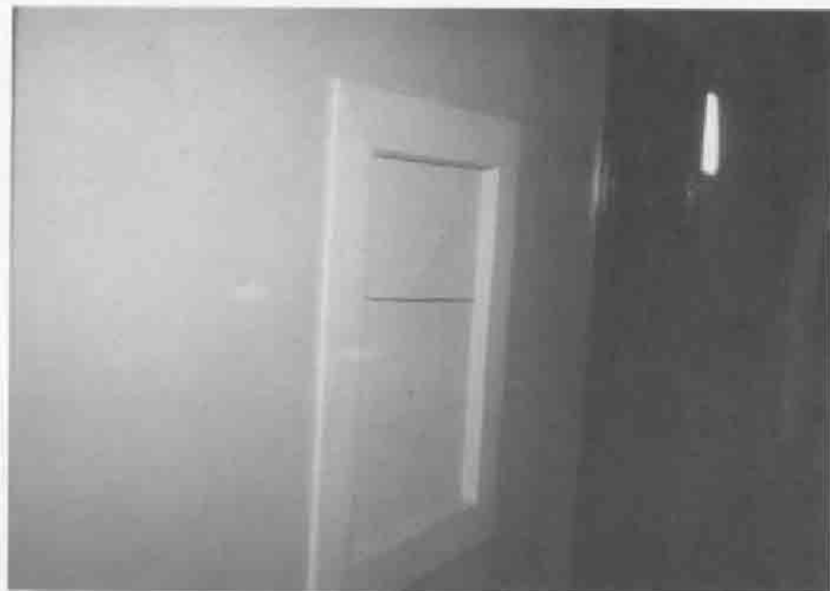
Typical Firebox Location in Hallway: Before Restoration
