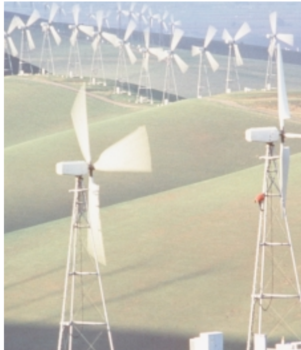
Wind power plant located in Altamont Pass near Livermore, California (photo courtesy of U.S. Windpower).
