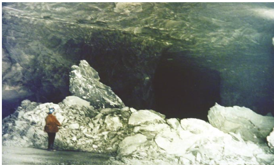
Figure 1. Large roof fall at underground limestone mine.
