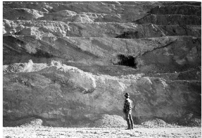
Figure 2.—Rock dump with 15-m-high vertical benches.
