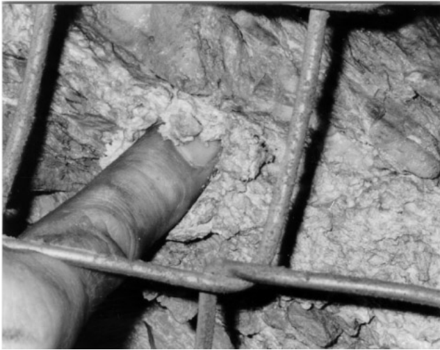
Figure 4. Soft, white gouge due to slip along argillite interbed
