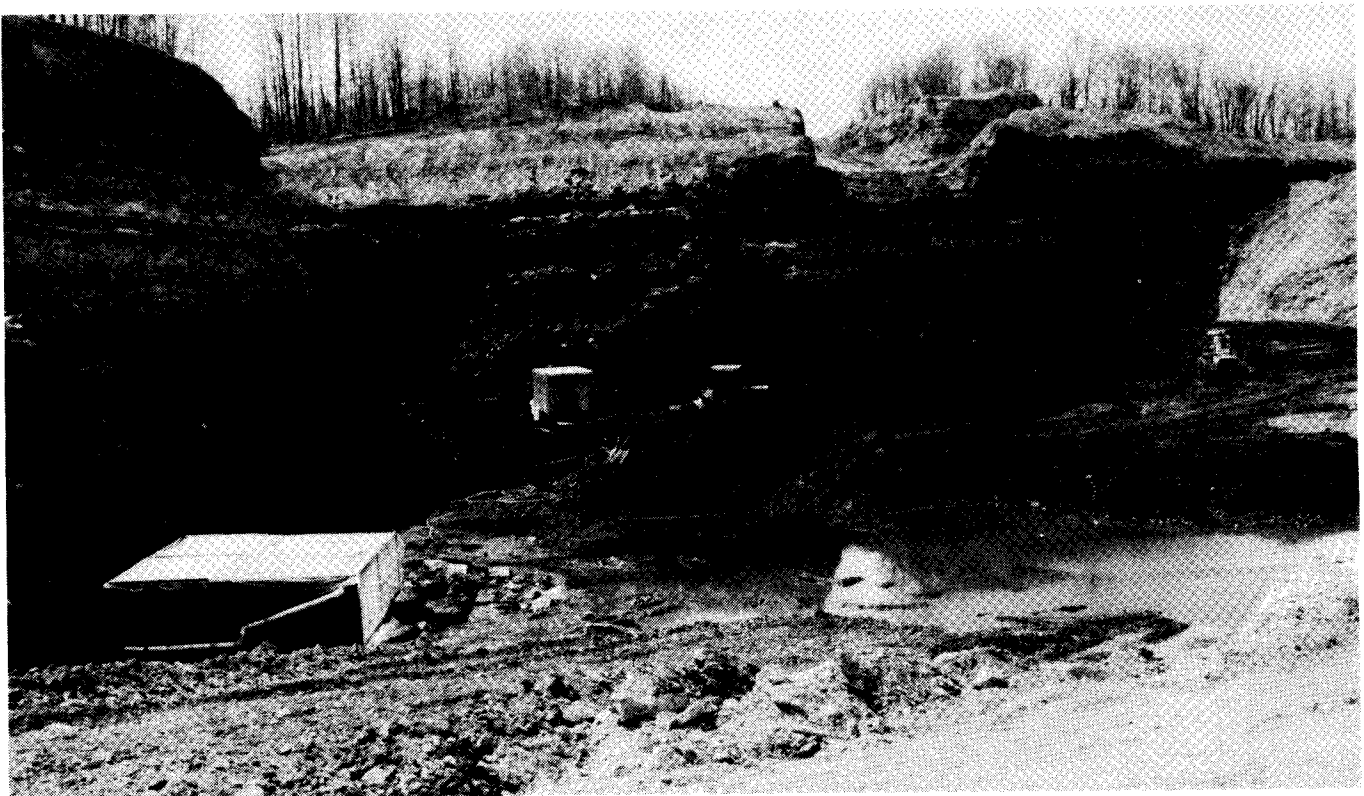
FIGURE 6. - Gallery in place against the highwall face. The instrumentation truck and connecting lines can be seen in the background.
