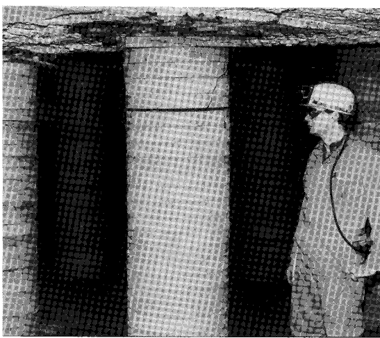
Figure 8.—Hydraulic flatjack arrangement in donut crib.
