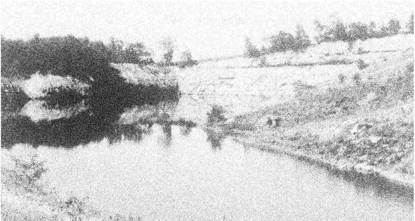
Example of abandoned unreclaimed surface mine exhibiting flooded pit, exposed highwall, and sparsely vegetated "dead" spoil.
