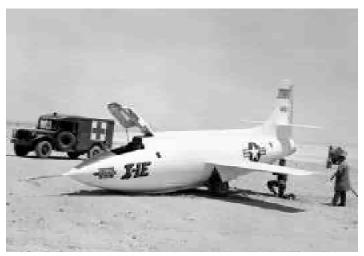
Photo E-2369. X-1E on lakebed with collapsed nose gear.
