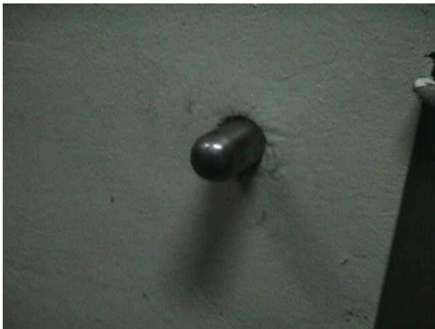
View of correct thermometer well
