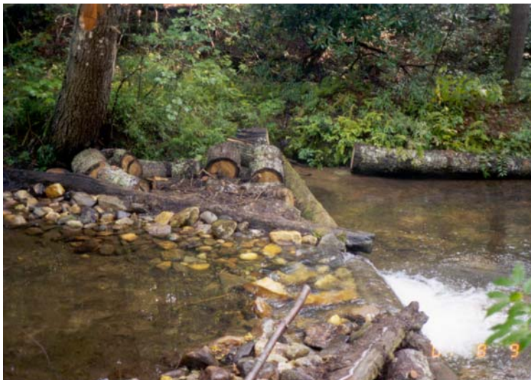
Repairs completed on a K-dam structure over thirty years old
