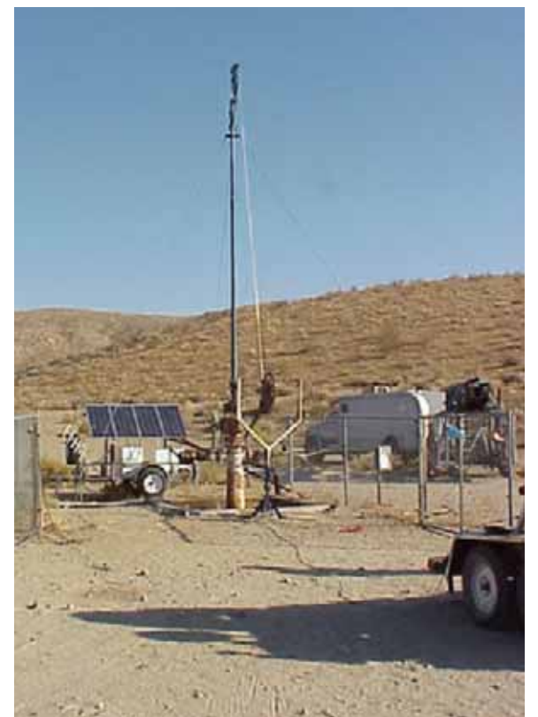
COSO — The US Navy's California geothermal well containing Sandia's hi-temp silicon-on-insulator tool. The solar panels are used to power the satellite transmitter and the tool located 3,100 ft below the surface.
