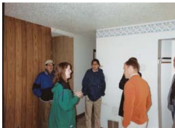
Touring a home abandoned due to mold.
