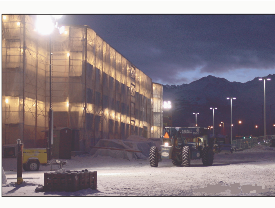
Photo 21: Cold weather construction site in Anchorage, Alaska
