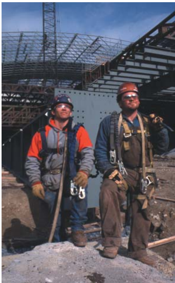
The OSHA Atlanta Regional Office is working with employers and employees to reduce fall hazards.
