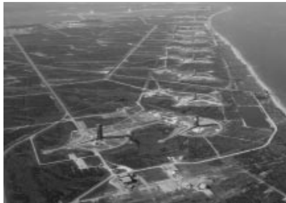
The two gantries of Launch Complex 36 (foreground), where Atlas rockets are launched, still stand on the easternmost point of Cape Canaveral. But the line of gantries extending north from the right-hand pad in this 1964 photograph have mostly been dismantled. Corrosion from the salt air had weakened the steel structures until they were no longer safe.
