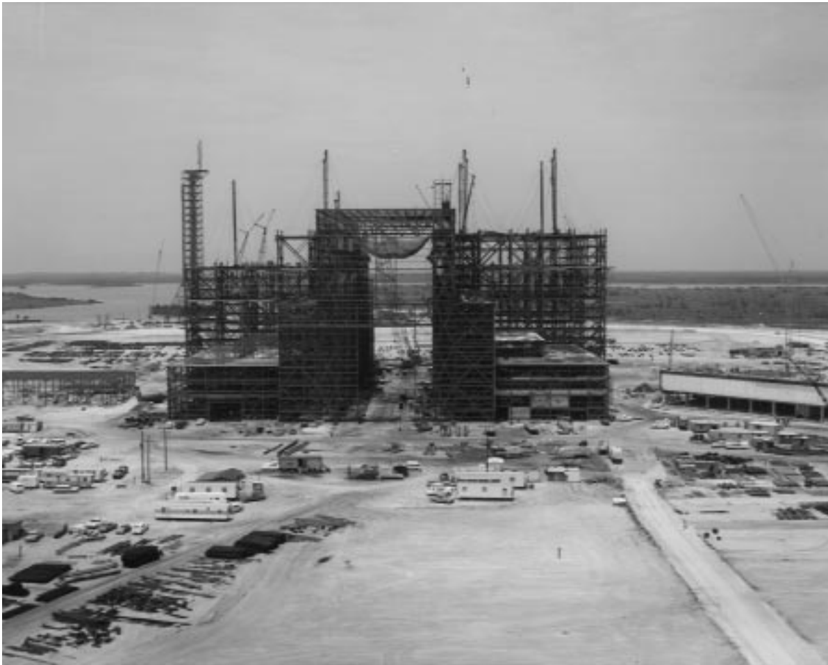
The steel framework of the Vehicle Assembly Building rises on Merritt Island during construction of America's Spaceport. The structure at right is the Launch Control Center
