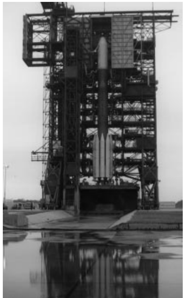
Protected by its gantry, a Delta rocket awaits launch under leaden skies at Complex 17. It later hurtled a GOES weather satellite into a geostationary orbit. Five of the Delta's nine strap-on solid booster rockets are visible in this photo.
