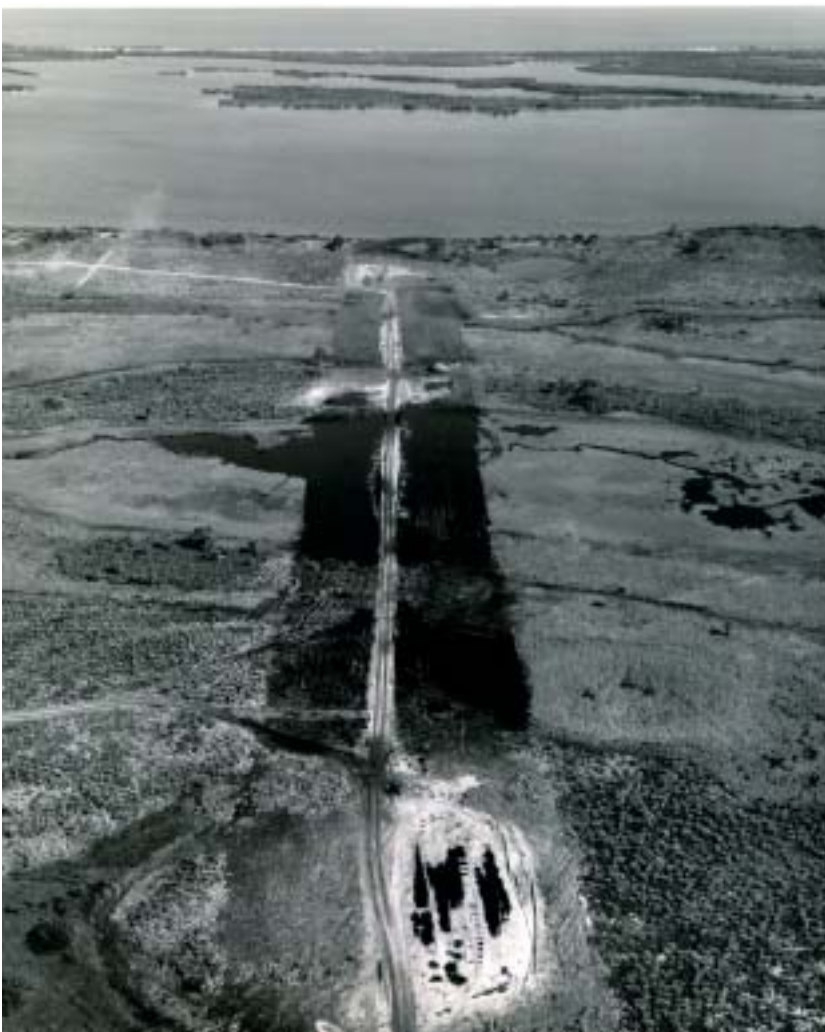
Aerial of the VAB site (foreground) and road to pad 39C (later pad A) during dredging of access channel, Jan. 23, 1963.
